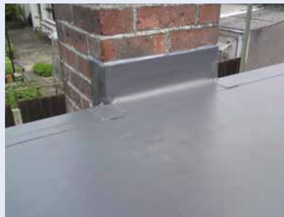
chimney flashing
